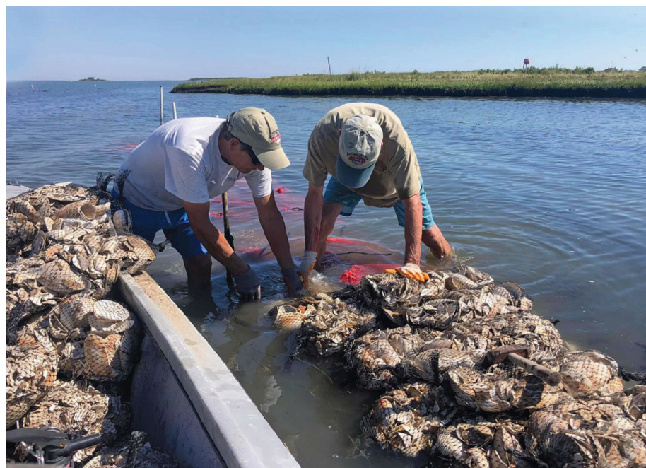
Shell bag deployment at Mordecai Island’s living shoreline.
